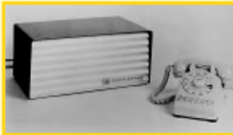
**1958** Bell's development of the modem data phone enables telephone lines to transmit binary data.
