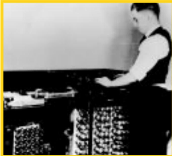
**1940** Konrad Zuse completes the Z2, which uses telephone relays instead of mechanical logical circuits.
