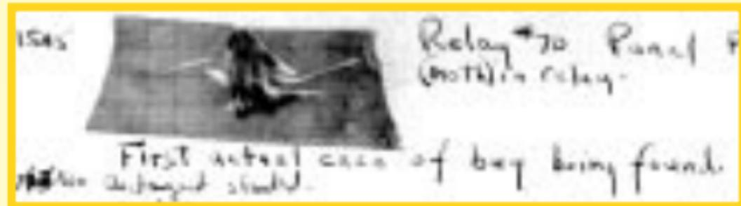
**1945** *Working on a prototype of the Mark II, in the summer Grace Murray Hopper finds the first computer "bug," a moth that had caused a relay failure.*
